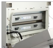
Redundant Exhaust HEPA Filters (Quantity 2)
