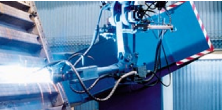
Robotic welding is used wherever possible to provide a high level of consistency and accuracy.
