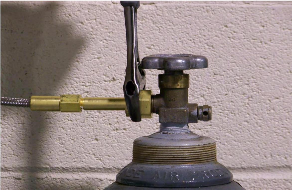
5. When replacing new CO2 tanks, use a CO2 compression disc or Teflon tape to prevent leaking.
