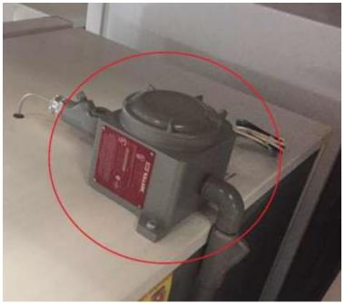
Mechanical Temperature Controller – located in the rear top location of refrigerator or freezer, inside of the metal enclosure.
