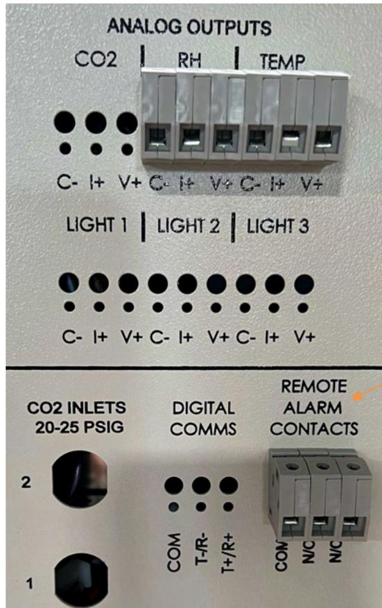
Remote Alarm Contact Connections
